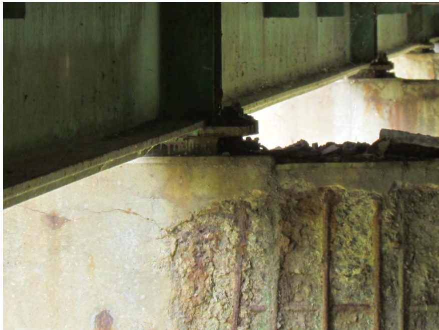
Photo 4: Bridge 1. View of concrete and debris accumulated on piers. Debris on beams from spider webs and bird droppings. No bat guano was observed.
