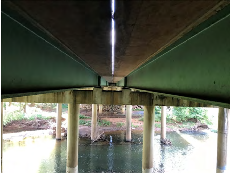
Photo 1: Bridge 1. View of expansion joint between lanes of Route 28 crossing Bull Run. Staining on piers appears to be due to runoff from road.
