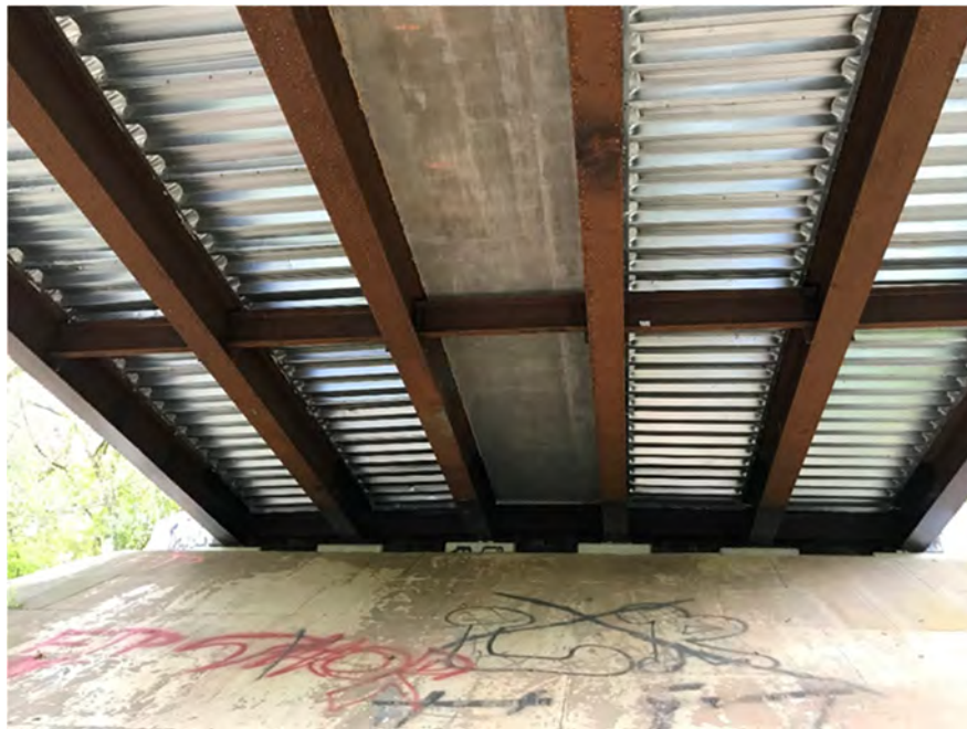
Photo 6: Bridge 2. View of abutment and steel decking. No visible staining or guano.
