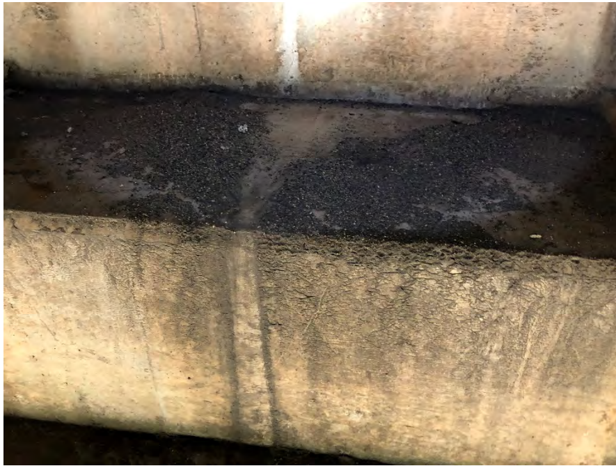
Photo 3: Bridge 1. View of water stains and accumulated sediment and gravel from road at the abutment. No bat guano was observed.
